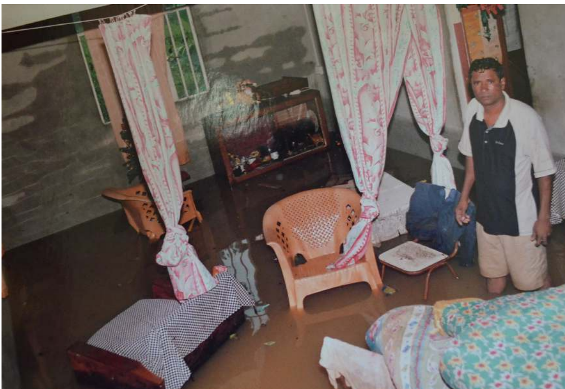
Mr. Toufoua in his living room during the 2015 aftermath of Cyclone Pam. The house was fully inundated and remained flooded for six days before the fire department pumped the mud and sediment from the house. All the furnishings had to be replaced.
